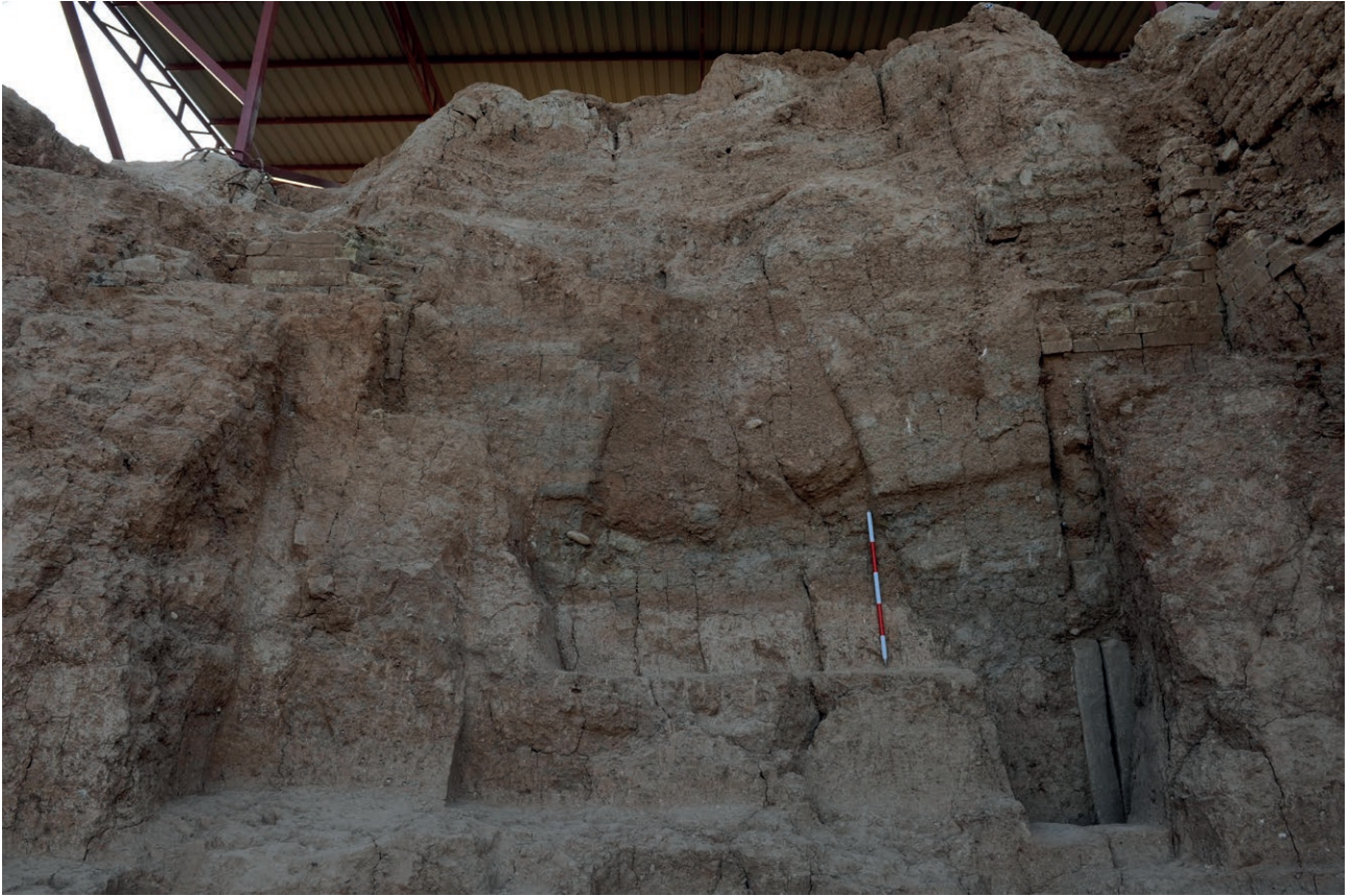
Fig. 15. The outer façade of the outer entrance of the Adad Gate in 2020, with the semicircular barrel vault and the narrowing corbelled arch. On the two sides, baked bricks courses can be noticed (photo by Serafino Rosso; courtesy of the Iraqi-Italian Archaeological Expedition at Nineveh).
