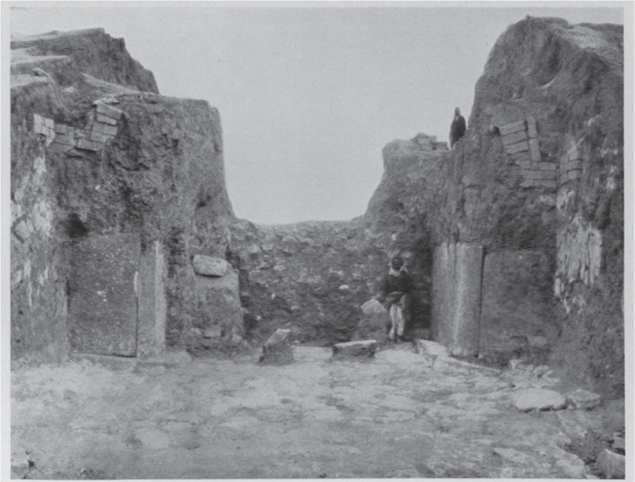
Fig. 25. Khorsabad. Gate 7, on the northern side of city walls, during the Oriental Institute of Chicago excavations, with plain orthostats and part of a baked brick archivolt on the upper part of the walls, on both sides (Loud 1936: 3).
