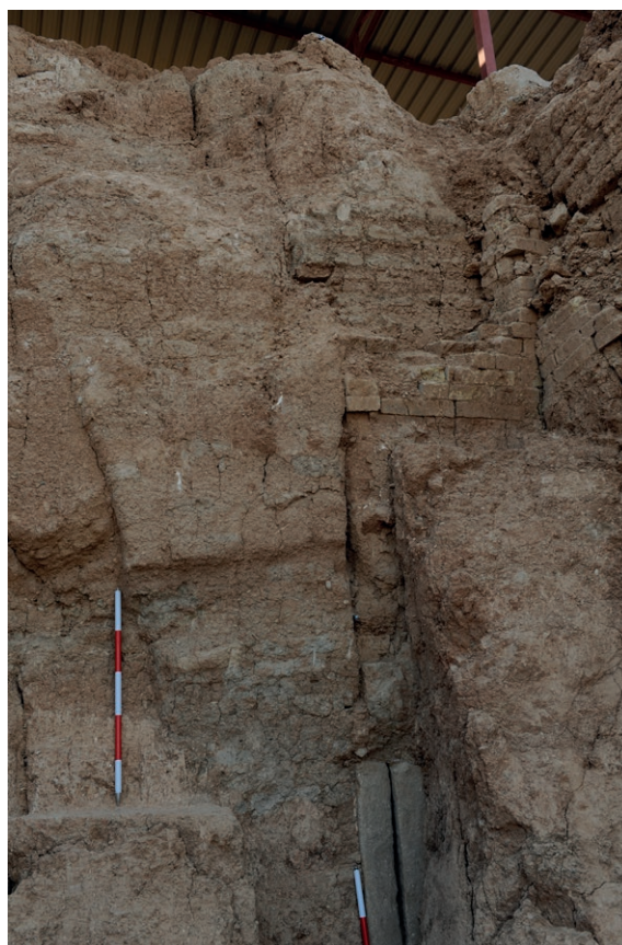
Fig. 19. Adad gate. Outer façade with baked bricks still in place on the upper part of the right-side mudbricks wall of the door, at the base of the arch. On the right, baked bricks still in place on the wall of the right side flanking tower (photo by Serafino Rosso; courtesy of the Iraqi-Italian Archaeological Expedition at Nineveh).
