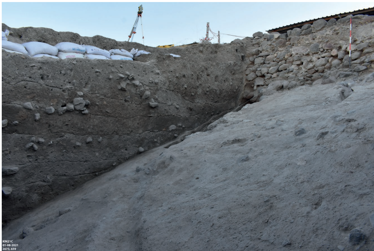
Fig. 6. Sector C3walls, rampart (Level C3walls.4), note in section the sequence of accumulations abutting the outer façade of the citadel walls (Level C3walls.3).
