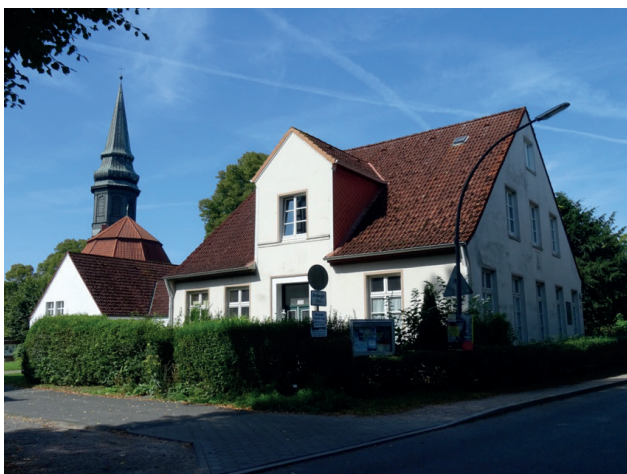
Figure 3 Parish Rectory in Billwärder, Hamburg, erected in 1840, in substitution of the old Rectory, where Runge was born in 1794 (Courtesy Billwärder Verein and Katja Haack, Hamburg)
