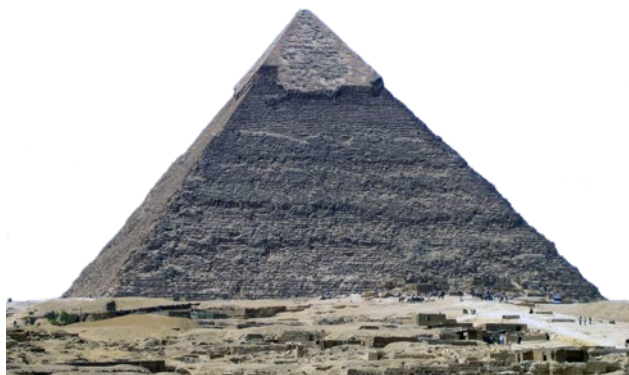
Figure 1. The Kephren Pyramid in which gypsum mortar was used.
