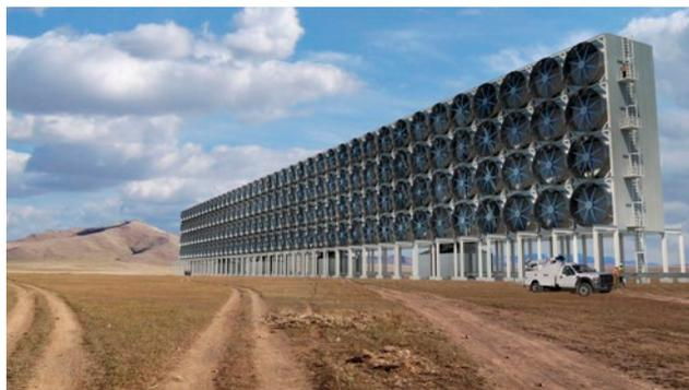
**Figure 5.** Proposed design to capture 1 million tonnes of CO<sub>2</sub> per year. Photo-illustration: courtesy of Carbon Engineering Ltd.
