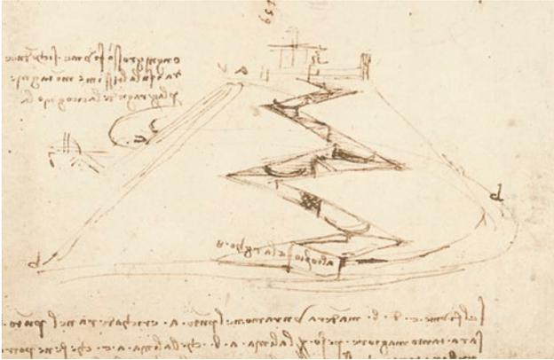
**Figure 21.** C.A., fol. 301 r, detail: big siphon to feed the highest navigation basin of a system of locks to bring boats up to the mountains.
