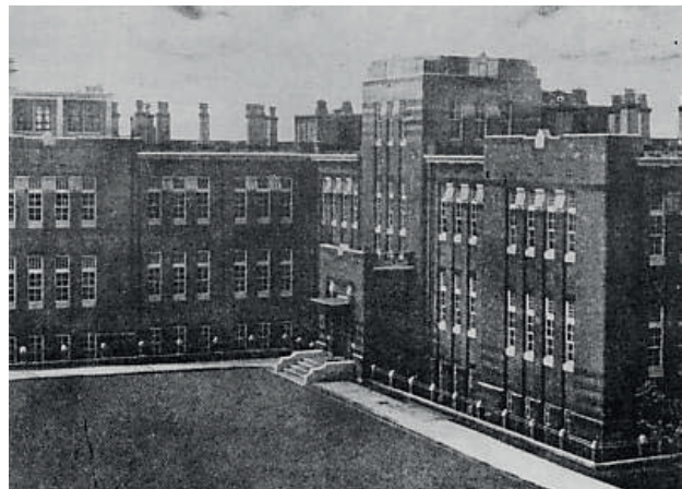
Figure 7. RIKEN building in Komagome, in northern Tokyo. (Reproduced with permission from RIKEN).
