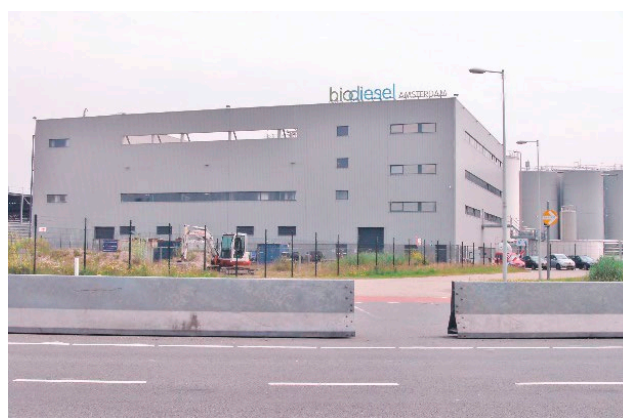
Figure 1. Biodiesel Production facility at Port Amsterdam.
