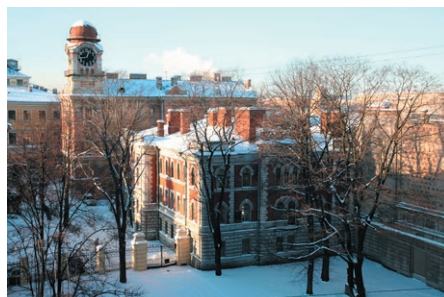
Figure 1. General view of the historic buildings of VNIIM, St. Petersburg, Russia, Moskovsky pr., 19. Photo from the collection of the Metrology Museum hosted by the D.I. Mendeleev Institute for Metrology, November 2010.
