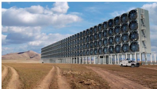
Figure 5. Proposed design to capture 1 million tonnes of CO 2 per year. Photo-illustration: courtesy of Carbon Engineering Ltd.
