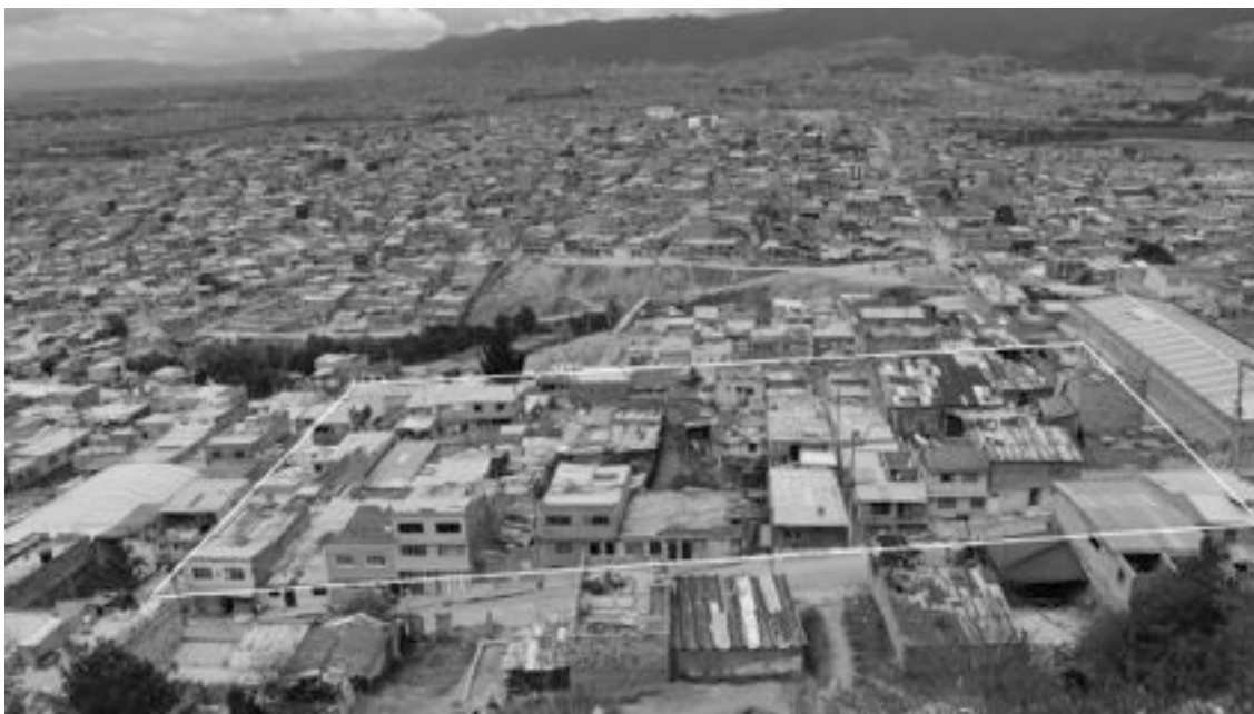
Fig. 6 - District Manitas, in Ciudad Bolívar. The pane highlighted two blocks that will be demolished for the construction of the station and facilities of ovovia. Photo: F.E. Forero Suárez
